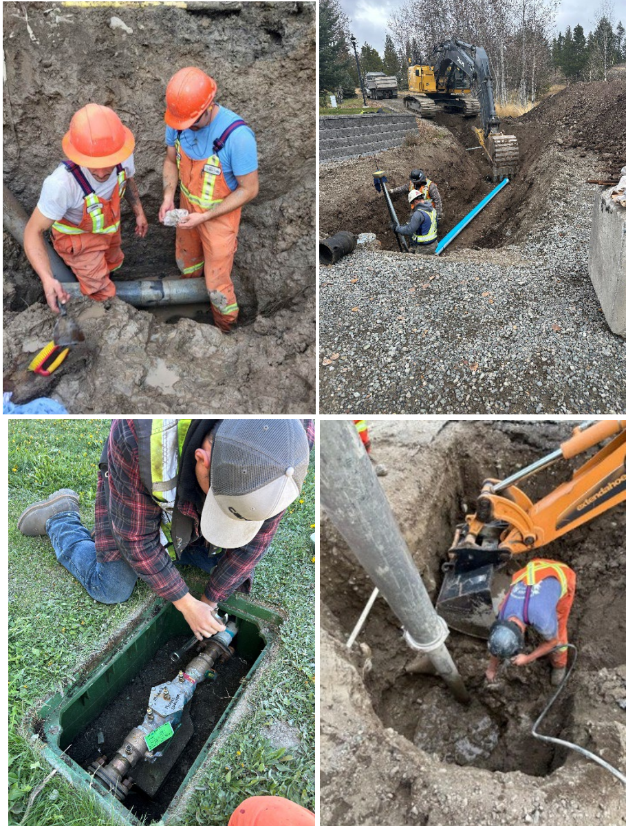
Figure 2: Water Main Repairs, Hydrant Maintenance and Flushing Program
