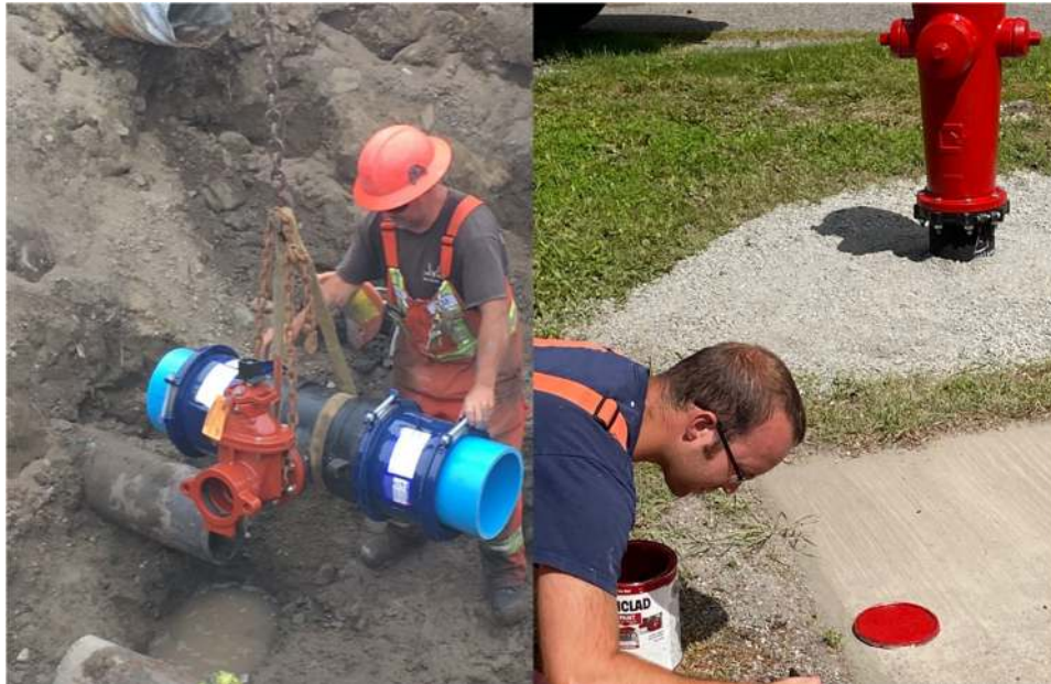
Figure 2: Fire Hydrant Extension and Water Main Repair
