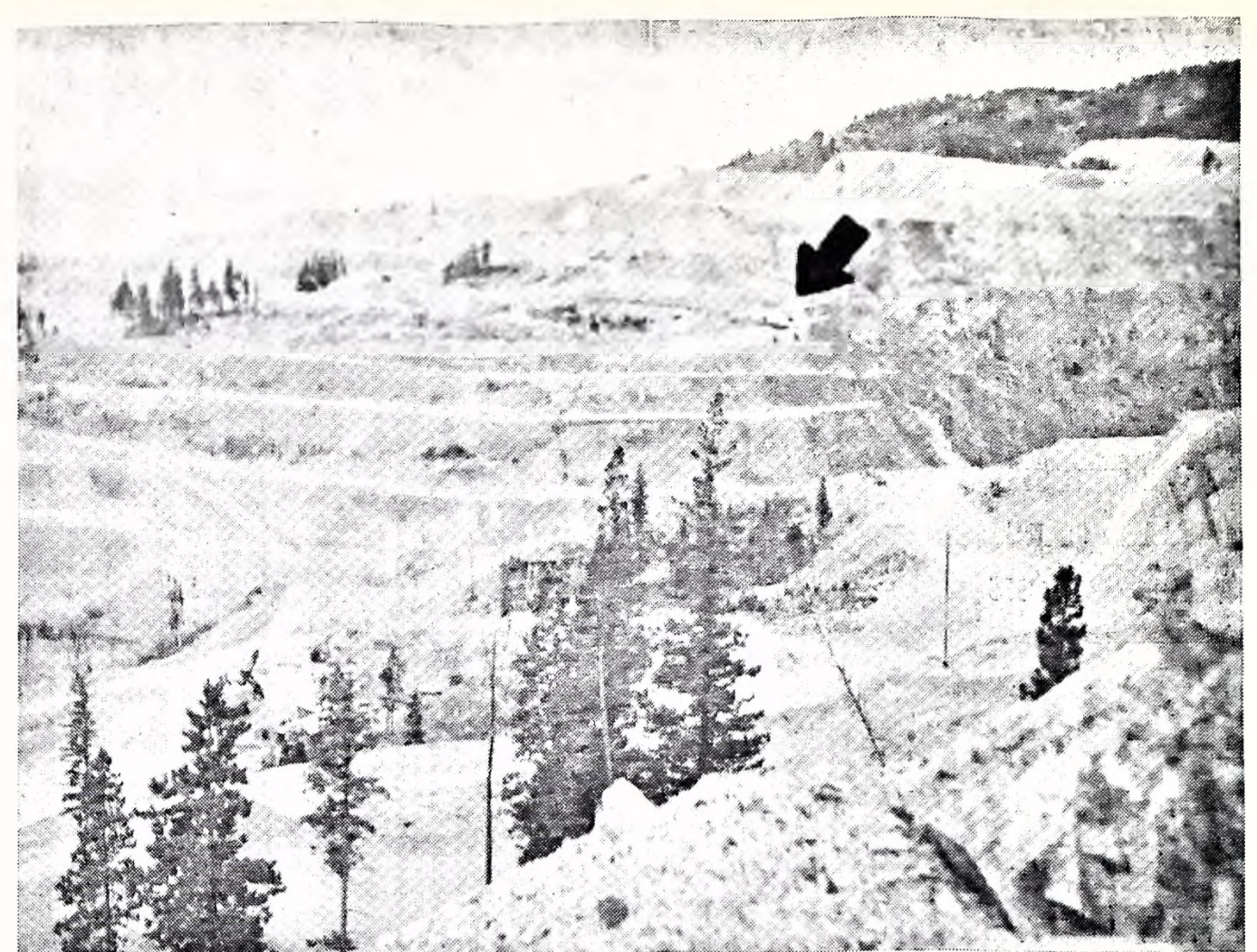
The arrow in the picture points to the small plane that did a big job in two days of flying at Craigmont Mines last Thursday and Friday. Here it is shown as it flies near the open pit area at one of the higher levels scattering a hardy grass seed over the ground. In the two days, 17,000 lbs. of seed, 65,000 lbs. of fertilizer were broadcast over 200 acres covering the waste dumps, open pit and lower face of the tailings pond. This is part of the long range program of land re-clamation started by Placer Developments at all their B.C. mines.
