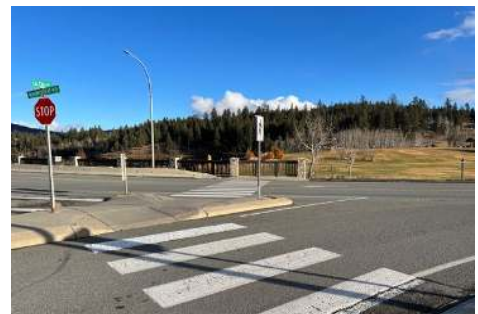
Figure 12: Crossing at Galena Ave.
