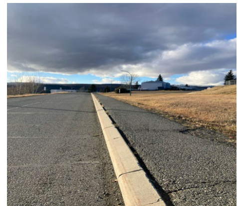
Figure 19: Asphalt sidewalk, District of Logan Lake, BC
