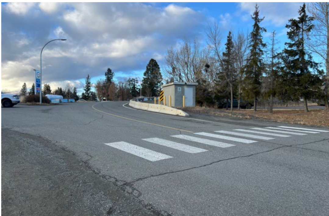
Figure 23: Crosswalk at Ponderosa Ave. in front of the Elementary-Secondary School
