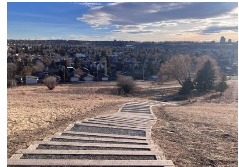
Figure 18: Example of a steep slope mitigation strategy at a park, Calgary, AB
