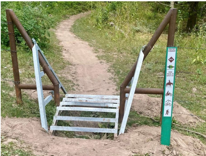
Figure 17 Example of a singletrack ride-over cattleguard.
