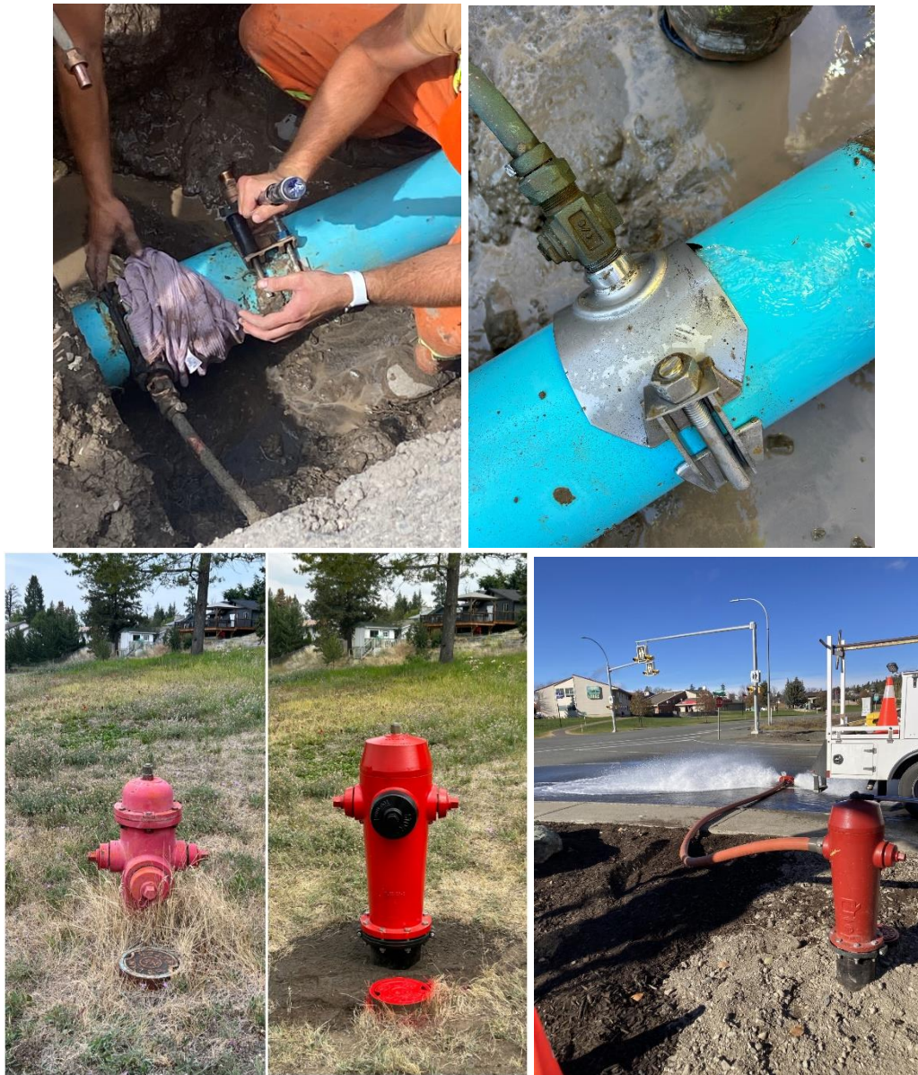
Figure 2: Water Main Repairs, Hydrant Maintenance and Flushing Program
